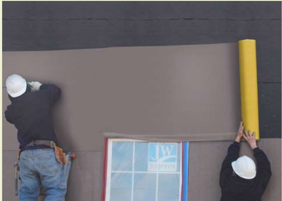
Home Slicker Stone & Stucco by Benjamin Obdyke is a 1/4"-thick 3D mesh material that has a fabric mortar block material over it. The 1/4" gap created by the 3D mesh creates the drainage space.
