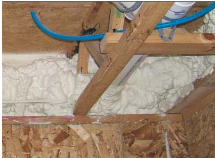
FIGURE 1. Fiberglass is not an air stop and cannot be relied upon to seal the rim joist (left). Best practice calls for sealing this area with spray foam (above).
