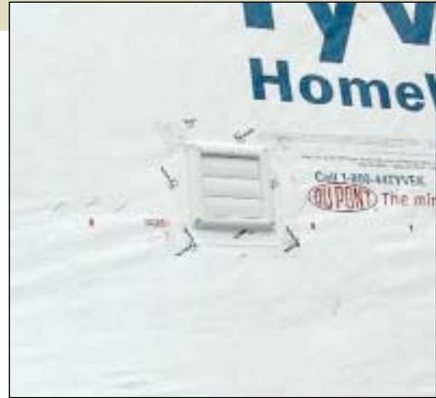
▼ **Overfastening.** Every staple through the water-resistive barrier is a potential water leak, so don't get trigger happy, as this installer did (below). In this case, water can actually be seen dripping off the ends of the staples inside the wall cavities (bottom). Best practice calls for a staple or cap nail every 12 to 18 inches along the vertical stud.
