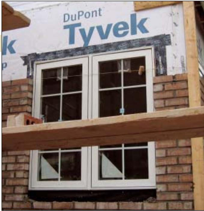
▲ **Improper head flashing.** The head flashing on this window is reverse-lapped with the housewrap. Before applying the head flashing, a flap needs to be cut in the housewrap so the head flashing can adhere directly to the wall sheathing and cover the nail fin. Once the flap is folded back down over the head flashing, water draining down the wall above the window will drain outside, not behind the head flashing.
