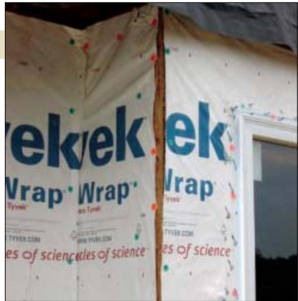
▲ Incomplete coverage. Water-resistive barriers must be installed correctly. The rips and gaps in the WRB shown here will allow any water blowing through to leak into the wall at the corners. The housewrap should be overlapped approximately 12 inches at the corners and sealed with an acrylic-backed tape. Note that the tape used for the window flashing is not an approved flashing material. It will probably fail as a result of differential movement.
