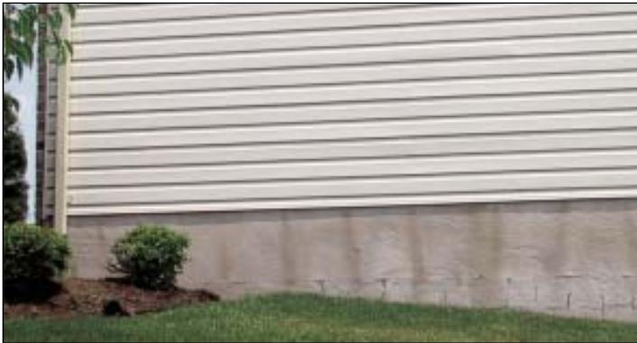
▲ Like all cladding, vinyl siding leaks. By design, it is made with weep holes to allow for drainage, but it needs a good drainage plane behind it to protect the wall. In this example, the secondary moisture barrier is doing its job, shedding enough water that wet spots are clearly visible underneath the vinyl siding.
