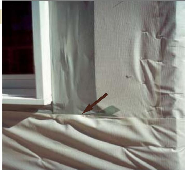
▲ **Reverse-shingled housewrap.** If you follow the arrow above, you can see that the secondary moisture barrier is reversed-shingled — the bottom layer overlaps the top layer, which means that any water that gets in behind the cladding can easily be funneled into the wall rather than draining away from it. When wrapping a wall, always start at the bottom so each successive layer overlaps the layer below.
