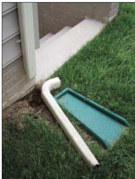
◀ **Maintaining drainage.** When I inspect a home for moisture problems, I look for signs of lack of maintenance. For example, here the downspout is disconnected from the leader, so all the water that runs off the roof is being funneled near the foundation. This can create a tremendous moisture load on the home.
