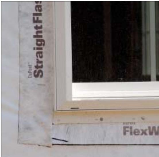
◀ **Proper window flashing.** The sequence of flashing a window is critical. Begin with a sill flashing that covers the rough sill and has a bottom flap that laps over the top of the housewrap as shown. This will ensure that any water that leaks through the window drains out. The jamb flashing should go on after the window has been installed, and should lap over the window flange to prevent wind-driven water from getting past the window into the rough opening.
