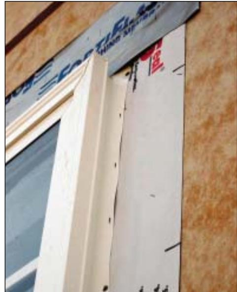
▲ **Why “splines” don’t work.** Applying jamb flashing before the window is installed meets the requirements of “Method B” of the ASTM window and door installation standard, but in my opinion it’s not the best way to flash a window. You can still end up with small gaps between the nail fin and the flashing as in this instance, which allow water to penetrate.
