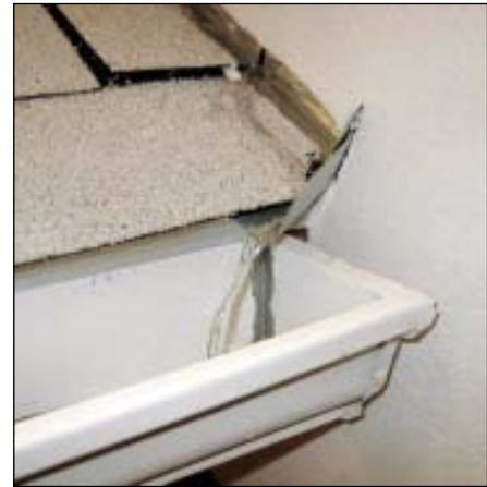
▲ **No kickouts.** The concentrated water flowing off a sloped roof can soak side walls (above left), concentrating the moisture load right at vulnerable window headers (not a great design). The solution is to divert the water away from the wall using kickouts — small pieces of sheet metal placed at the end of the step flashing and sealed to the wall and roof sheathings with some peel-and-stick flexible flashing (above right).
