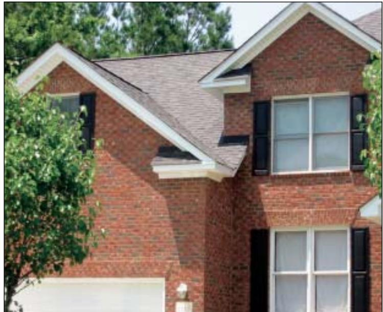
▲ **Design solution.** Here's one example of how to detail intersecting roofs to avoid a horizontal valley. By keeping the gable ends on different planes, the valley is allowed to run unbroken, so water can drain away freely.
