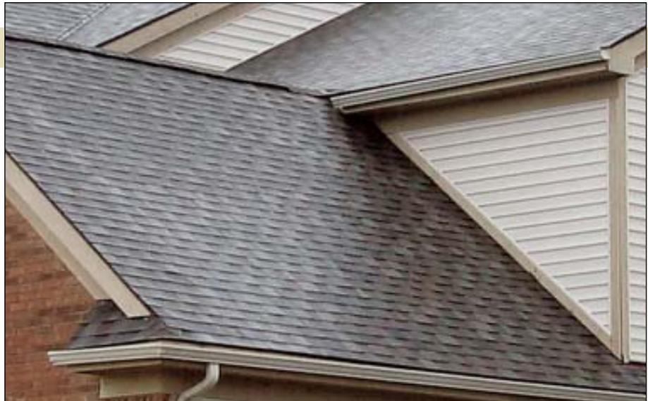
▲ **Ridge intersecting eaves.** The problem with this design is that all the water that runs off the higher roof is collected into the gutter. Note that there is no downspout, so all the water that runs off the higher roof runs toward the poorly flashed ridge cap of the intersecting roof. The solution is to drop the ridge so the eaves and the gutter of the higher roof can run uninterrupted above the lower roof ridge. And, of course, pitch the upper gutter to a downspout at the corner.
