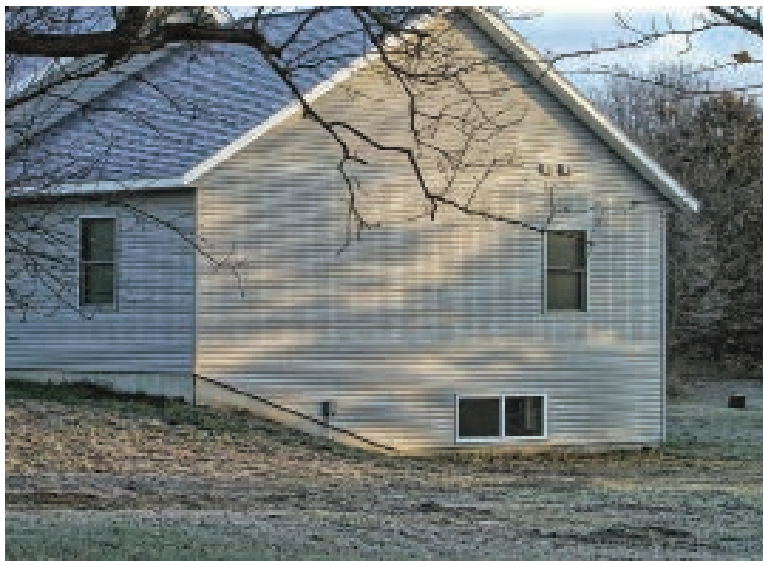
Studs conducting heat (above left) stand out on a frosty morning. Exterior insulation would eliminate this heat loss. Air-sealing is critical when walls are vapor-closed to the outside. Here, a builder has correctly air-sealed a bottom wall plate (above right).
