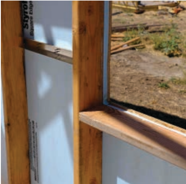
Sheathing can be applied outboard of the foam (above left). This lets the sheathing dry to the outside. ThermalBuck (above right), an insulated window mounting system, creates a positive attachment for the window while limiting thermal bridging.
