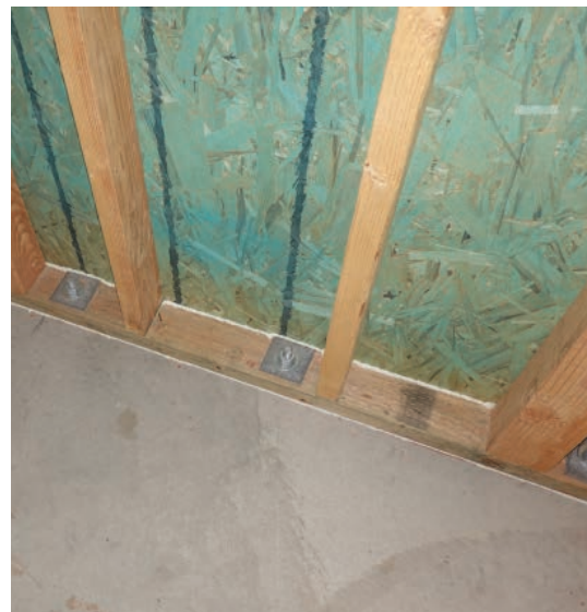
Studs conducting heat (above left) stand out on a frosty morning. Exterior insulation would eliminate this heat loss. Air-sealing is critical when walls are vapor-closed to the outside. Here, a builder has correctly air-sealed a bottom wall plate (above right).
