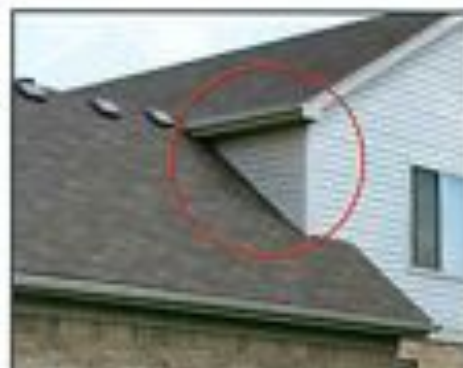
Photo 3 - Ridge intersecting eaves.
