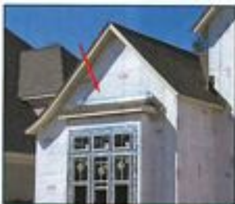
Photos 13 and 14 - Reverse-shingled weather barriers.
