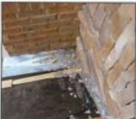
Photo 12 - Metal flashing reverse shingled over brick.
