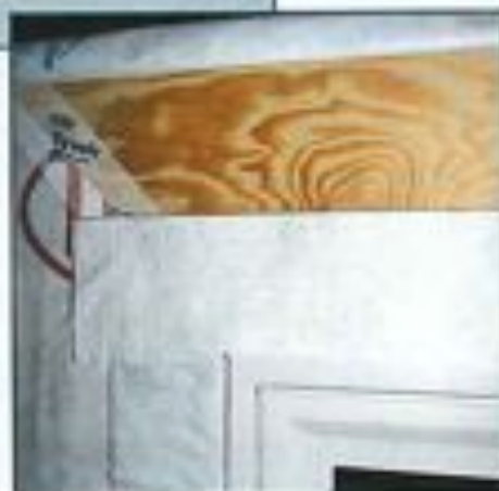
Photo 29 - Head flashing attached from nail fin to sheathing.
