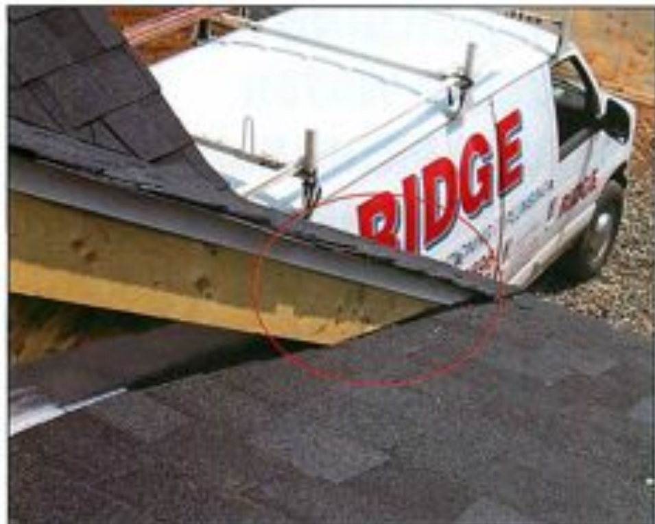
Photo 4 - Intersecting roof plane.
