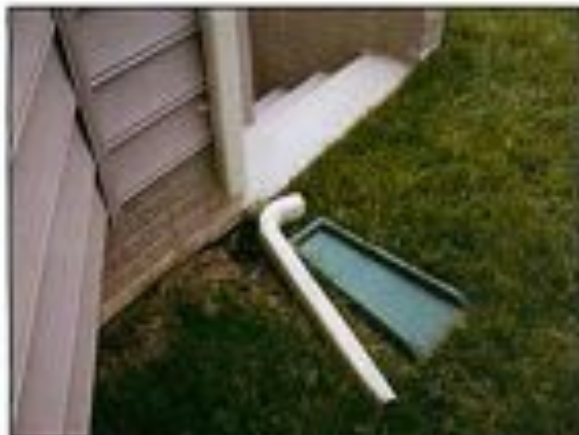
Photo 34 - Disconnected downspout.
