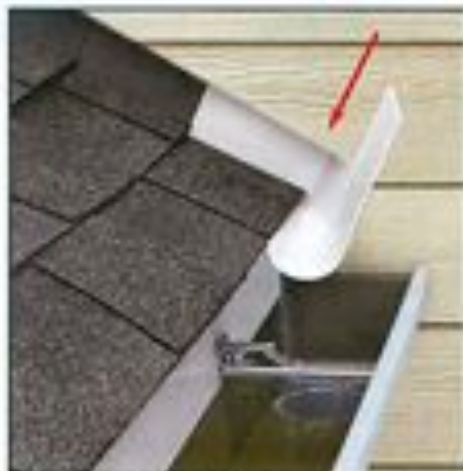
Photo 11 - Premolded kickout flashing (courtesy DryFlikt.com).
