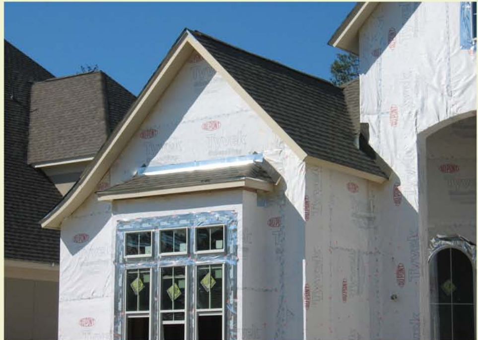
The head flashing of this window (as well as the bay roof area) is reverse shingled. If water gets behind the wrap it will enter the home at the window header.
